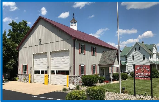
Figure 125 Union Fire Company No. 1 of Oxford substitution in West Nottingham Township.
