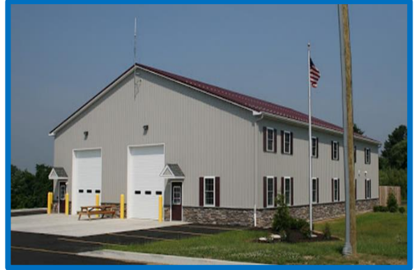
Figure 126 West Grove Fire Company station in London Britain Township.
