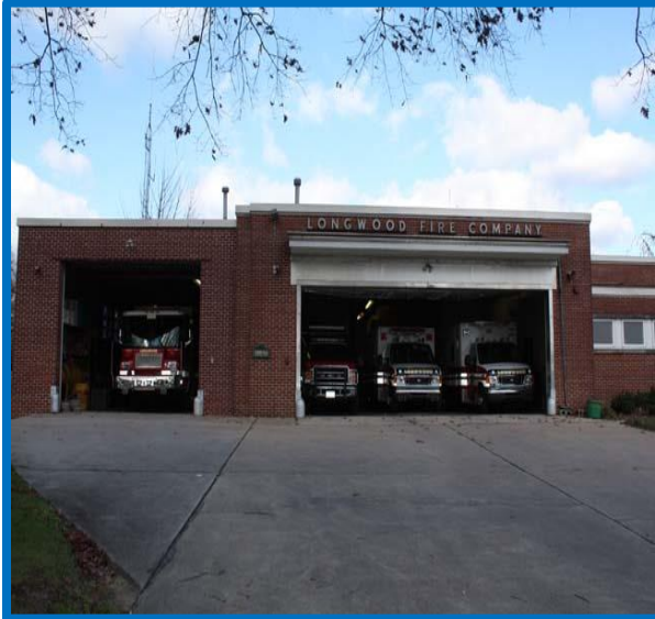
Figure 113 Longwood Fire Company Front View
