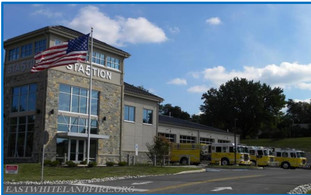
Figure 121 East Whiteland Fire Company's new station opened in 2015.
