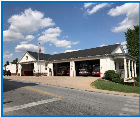
Figure 107 Union Fire Company No. 1 Front View with Upper Fire Apparatus Bays
