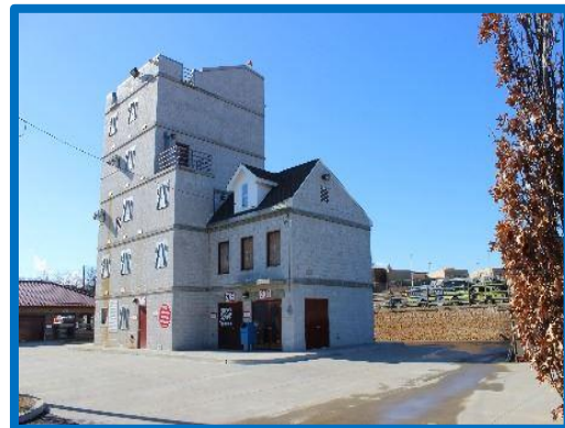
Figure 145 Drill Tower/Scenario Building
