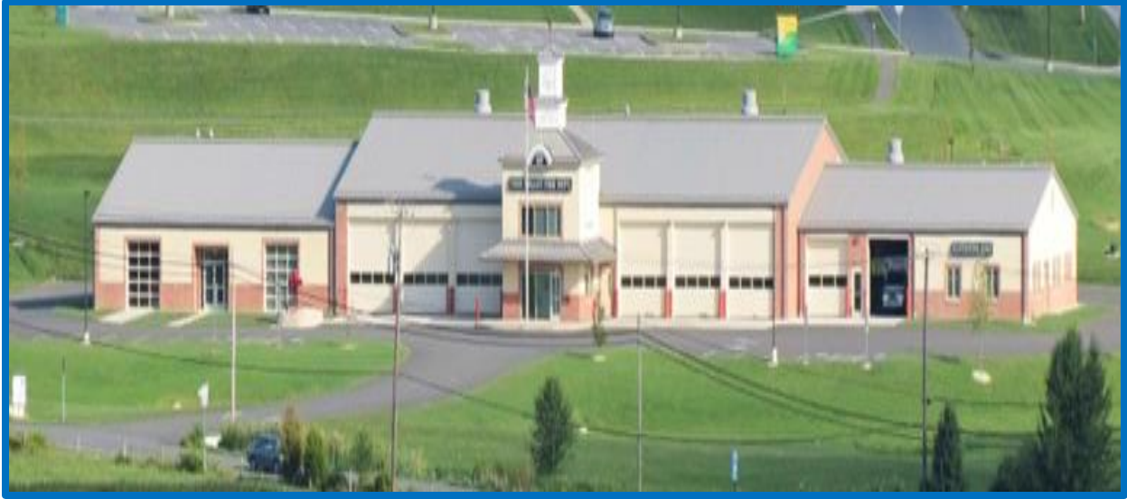
Figure 122 Twin Valley Fire Department's new station opened in 2009. Elverson-Honey Brook Area EMS and a Brandywine Hospital medic unit also operate from this multi-functional facility.
