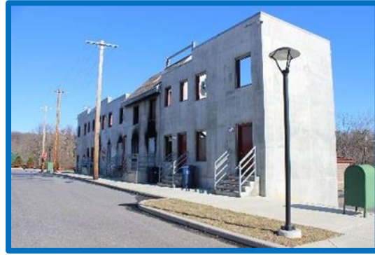
Figure 150 Tactical Village/Burn Building
