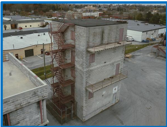
Figure 156 West Chester Fire Department Training Center Drill Tower
