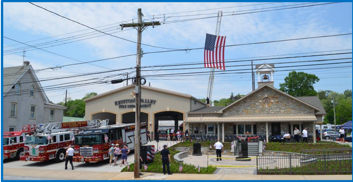
Figure 124 Keystone Valley Fire Department's existing station was extensively renovated and updated to meet the department's evolving needs.
