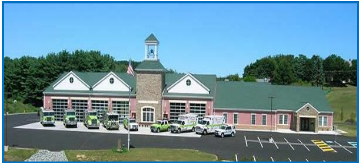
Figure 123 Avondale Fire Company's station opened in 2007. This station also serves as both fire and EMS deployment locations with the fire company operating BLS ambulances and Southern Chester County EMS responding with a medic unit.
