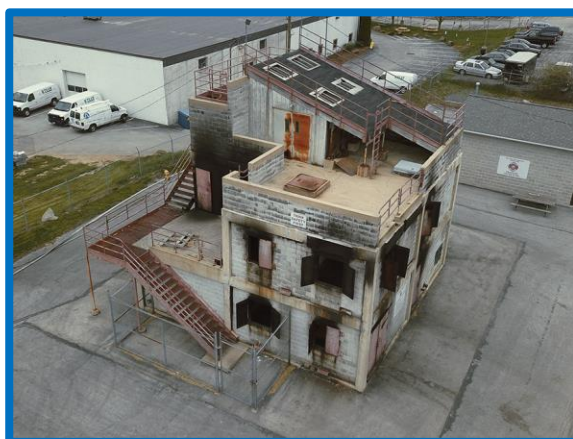
Figure 157 West Chester Fire Department Training Center Burn Building
